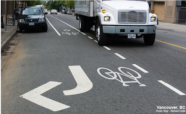
Bike lane with turning arrow and dashed striping at intersection
