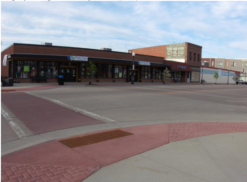
Street View of Site 1 existing buildings along 2nd Street (2020)
