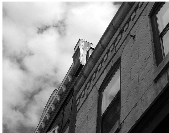
Historic rooflines include corbels of stone and brick, parapets of stone, brick, metal, or wood, and a variety of other decorative features.
