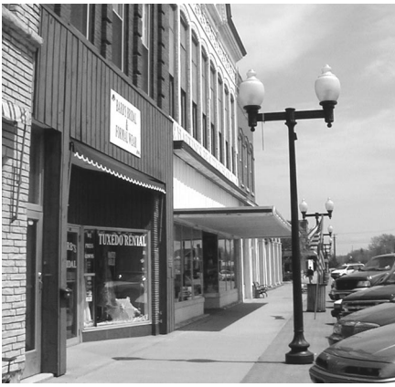
Historic features are probably hiding behind the covered-over facade at left.
