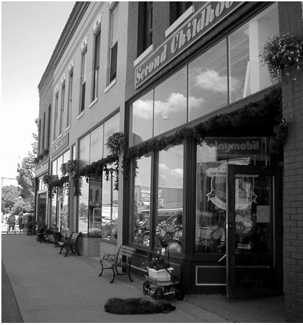
Signs like that at upper right occupy the signband area of the facade and do not detract from the historic character of the building.
