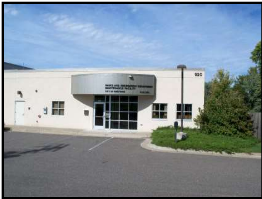
Joint Maintenance Facility
