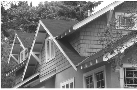
New roofs and dormers should be carefully designed to be compatible with the existing building.
