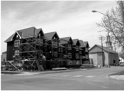
New housing under construction at Guardian Angels, 2002.
