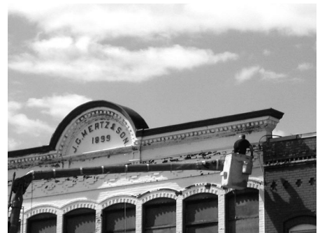
J.G. Mertz & Son Building (1899) during restoration, 2002.
