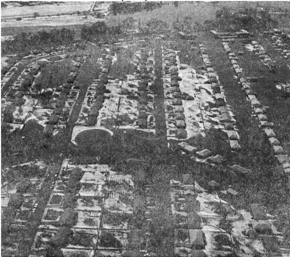
Figure 11a. Floodwaters from Vermillion River north of Linear Park. Hastings Gazette reported this on Dec 20, 1965: “Looking south, this airview of Westwood Addition shows the area hardest hit by flooding from the Vermillion River. The river itself, normally a quiet stream only a few feet wide, runs along the top of the picture, with trees outlining its natural course. Photo was taken on Wednesday, April 7, when the floodwaters were still holding after the crest. West 19 th Street curves across the center of the picture. The outline of the hockey rink in the West 19 th Street Park can be seen at left center. A total of 42 blocks in the city were under water from Monday through Thursday of that week, and more than 250 families were forced from their homes.” Photo from Pioneer Room.
