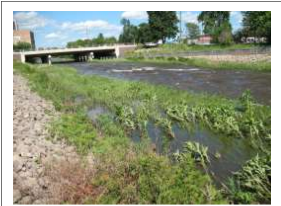
Photo 16. View looking east towards Hwy 61 bridge. Note the riprap on both sides of the channel. Vegetation is a mix of native and non-native (cup plant in middle foreground and reed canary grass in background).
