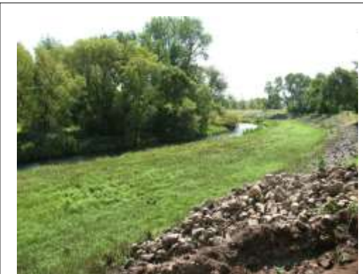
Photo 13. West end of property, west of river bend. Note the mowed vegetation near the river and the riprapped bank.
