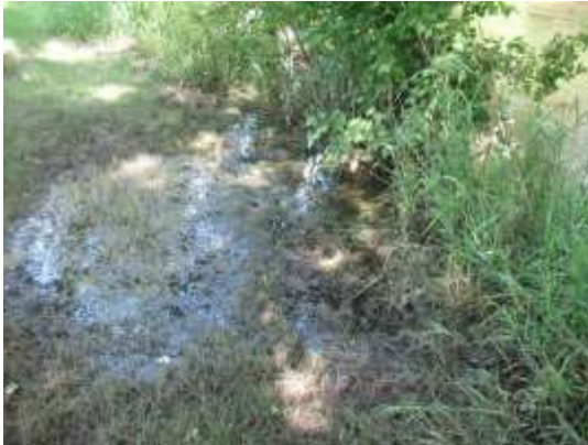
Photo 33. Flooding onto the mowed turf buffer. The area of flooding actually extended farther upland: note the brown stains on the grass from river sediment.
