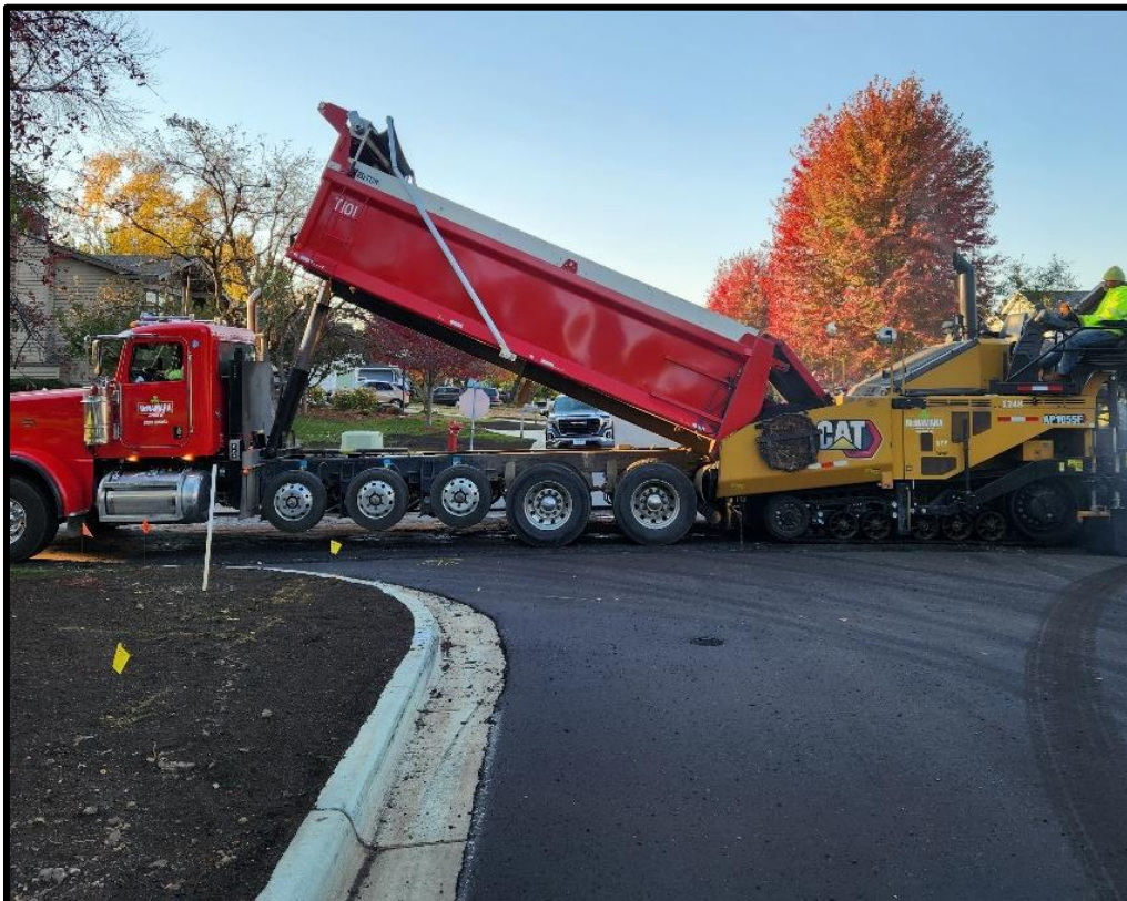
Final Street Paving
