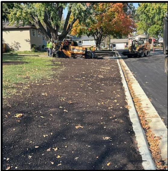
Final paving of driveways and streets
