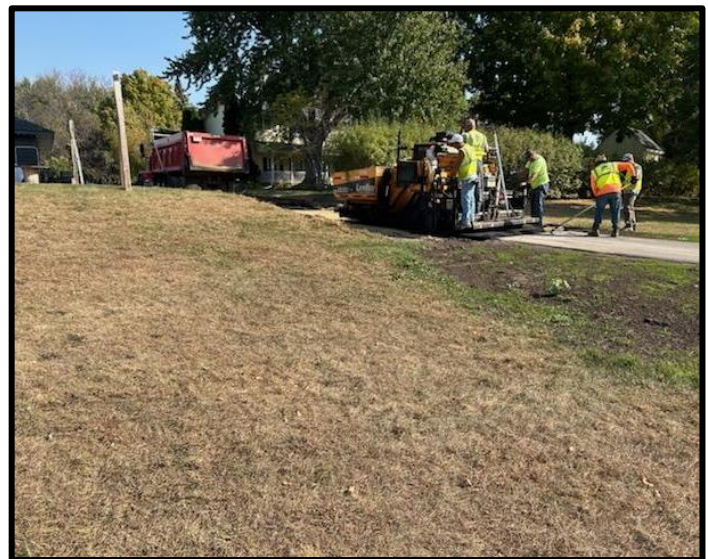
Paving of Pleasant Park Trail
