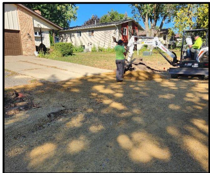
Driveway preparation for Concrete
