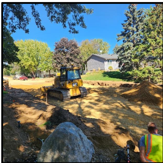
Road preparation for concrete and paving
