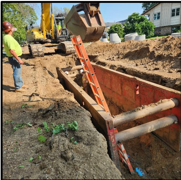
Water main improvements
