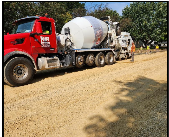
Concrete curb and gutter replacements
