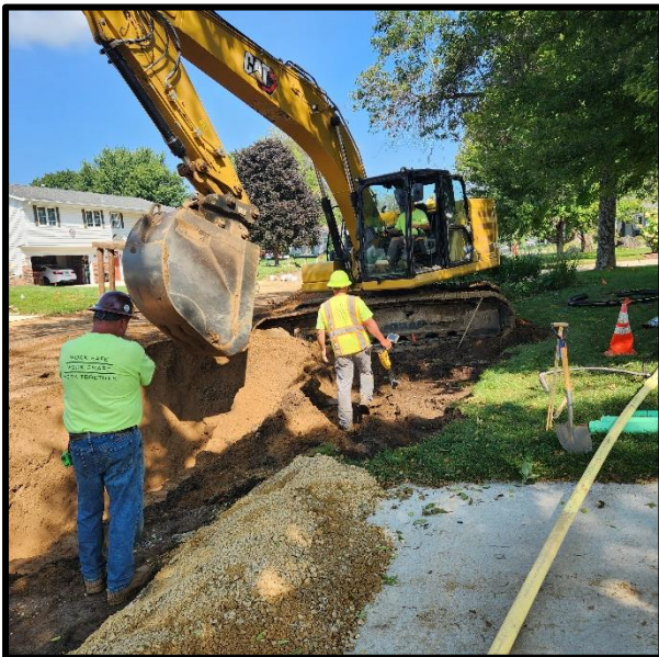
Sanitary and water service replacements
