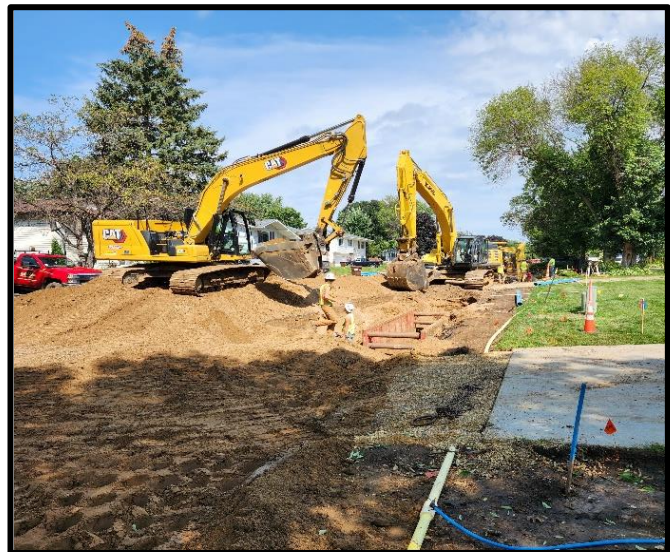
Water main improvements
