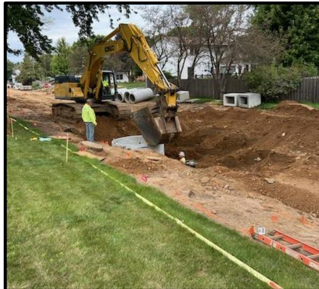
Storm sewer improvements
