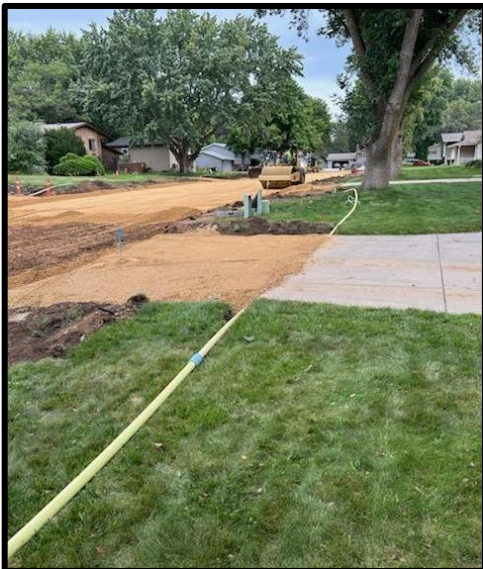
Grading of road base material
