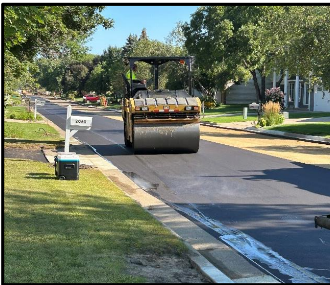
Paving of Highland Drive
