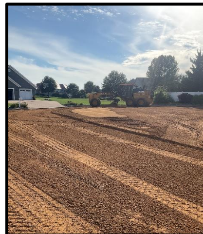
Road base material preparation
