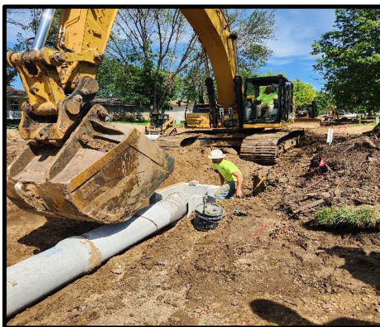
Storm sewer improvements
