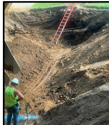
Water service installation
