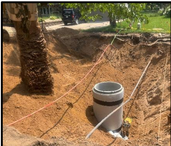
Sanitary sewer improvements
