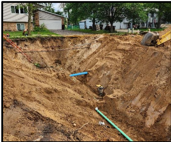
Sanitary sewer and water service replacement
