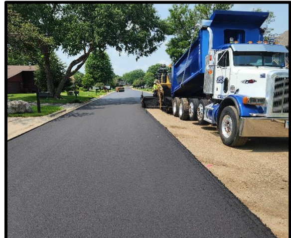
Street paving on 21 st Street
