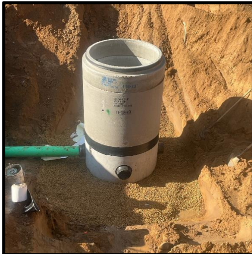
Sanitary sewer improvements on 17 th Street
