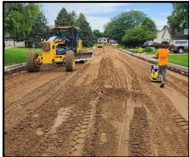
Street grading on 21 st Street
