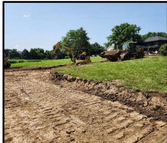
Trail reconstruction at Pleasant Park
