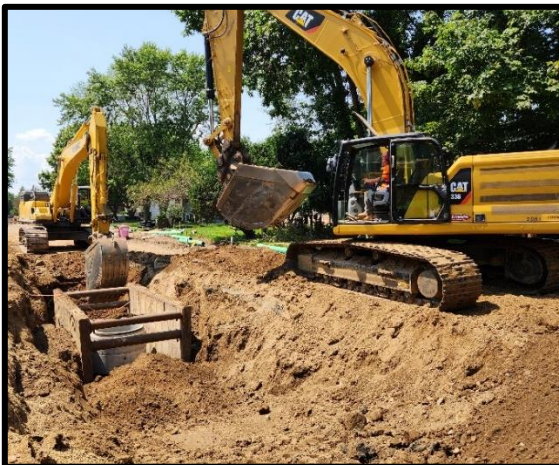
Sanitary sewer improvements on 17 th Street
