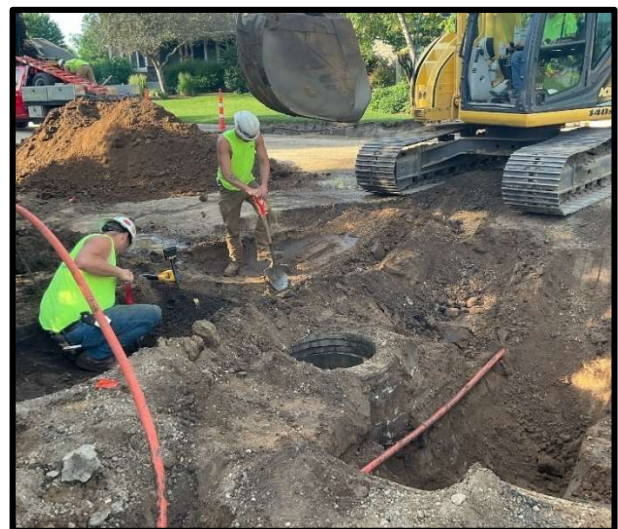
Storm sewer improvements on Brooke Ln
