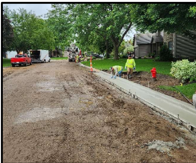
New curb being poured along Brooke Ln
