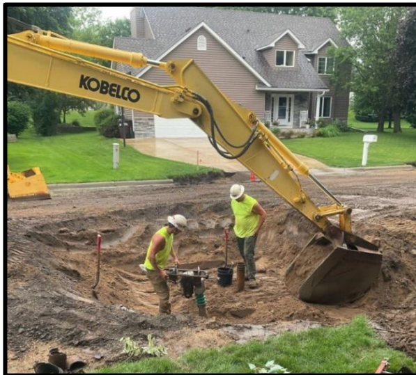
Compacting around rehabilitated water valve
