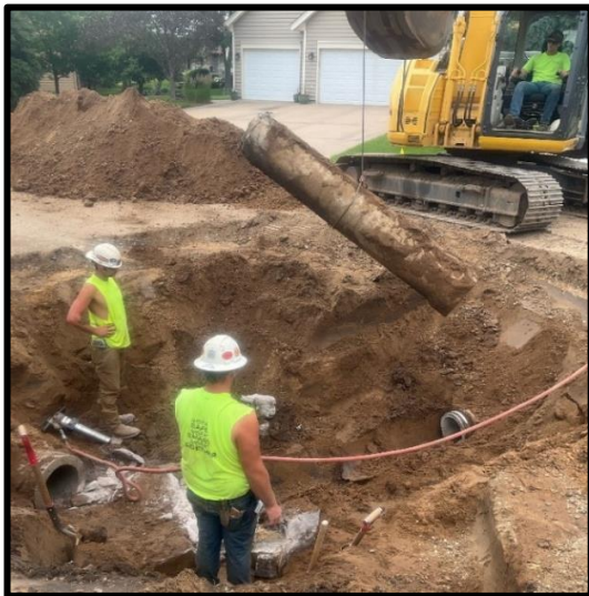
Removal of existing storm sewer
