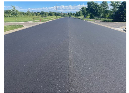
Right: Paving Complete
