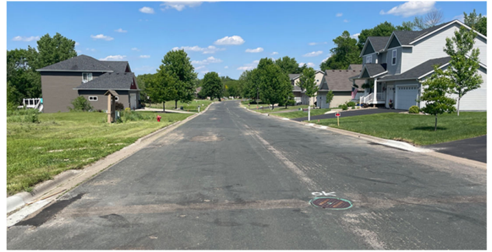
Above Right: Curb replacements on Bohlken Dr
