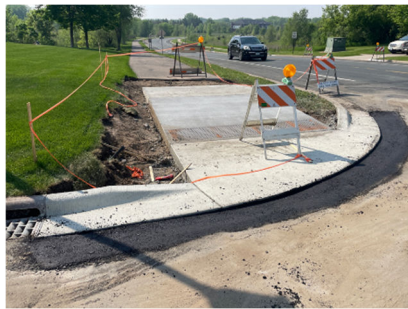
Above Center: Patch bituminous around curb & gutter
