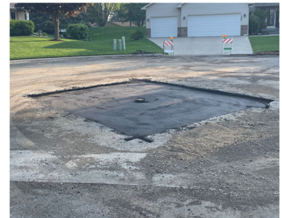
Above Right: Patch bituminous around gate valve
